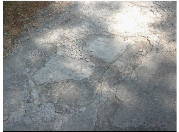
Cracking/displacement @ driveway
