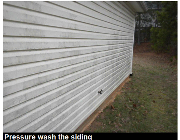
Pressure wash the siding
