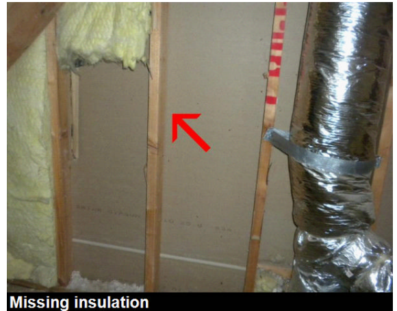
Missing insulation
