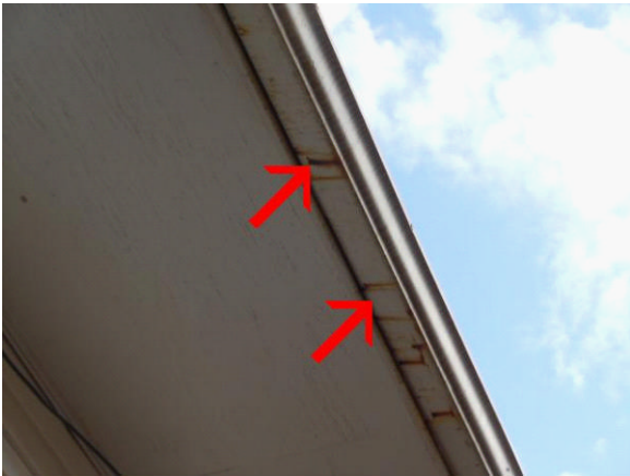
Rusted gutter
